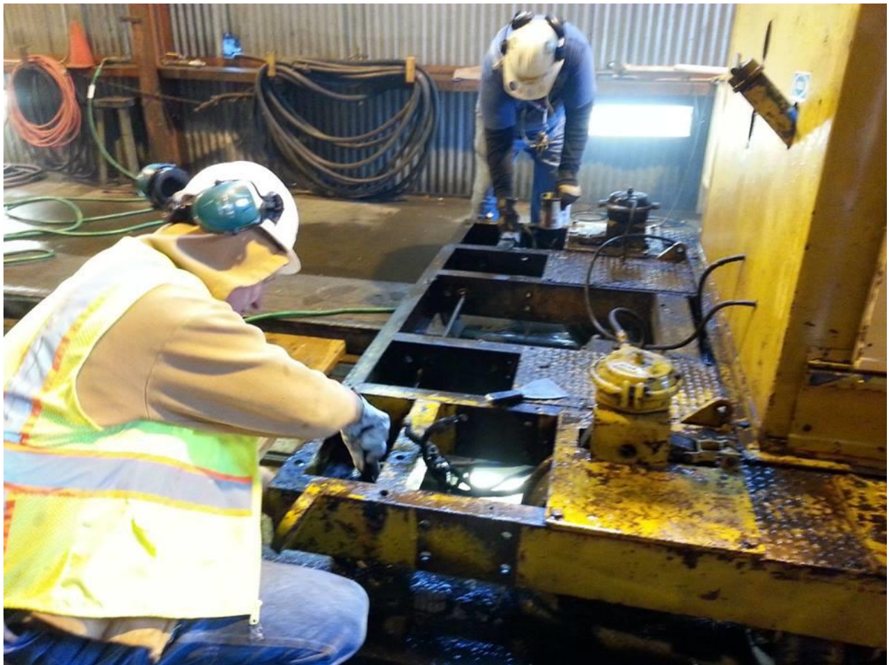
Now that they can see things, Steve and Mike F. are able to remove more components of the hydraulic system
